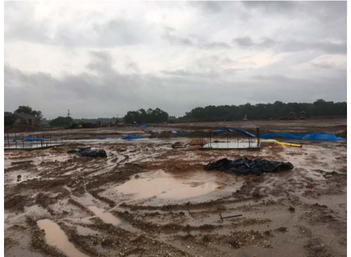
10. Ticket / Entry slab on grade
