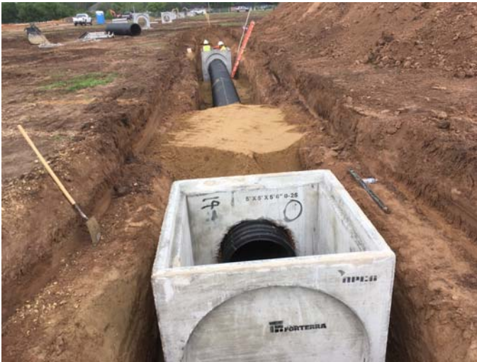
7. Storm sewer installation at home parking
