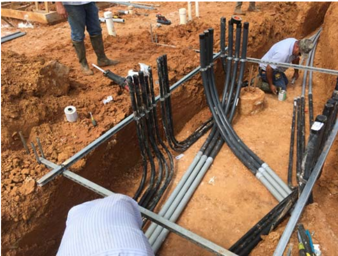
13. Underground electrical at concessions
