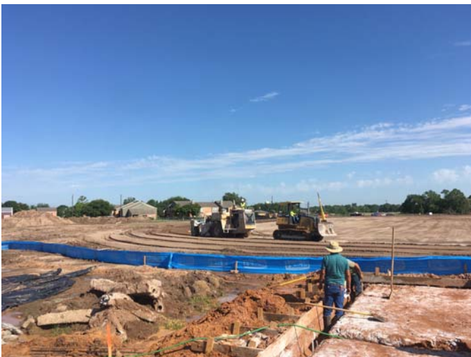
11. Remix of lime stabilization at field
