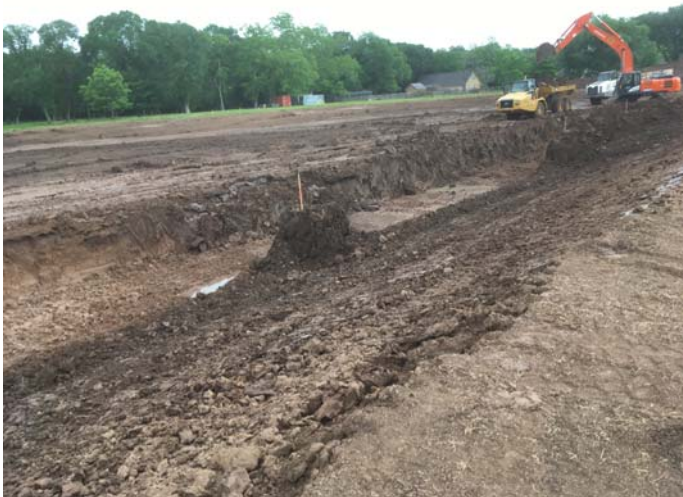
3. Detention pond excavation
