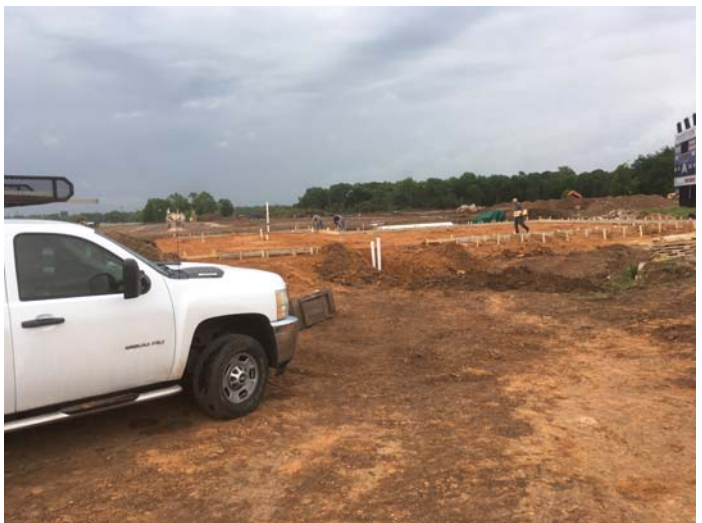
6. Concrete formwork at concessions building
