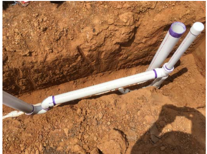
2. Underground plumbing installation at concessions
