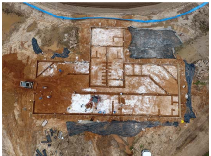
18. Grade beam excavation at concessions
