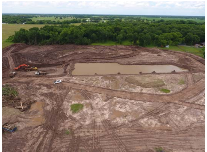
16. Detention area after multiple rains (5/14/2019)
