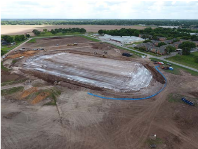
1. Lime stabilization of field subgrade
