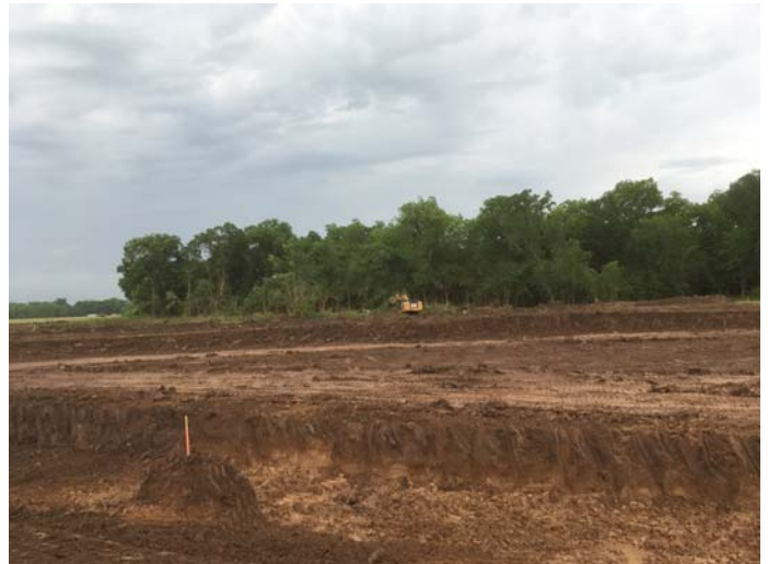
4. Detention pond excavation
