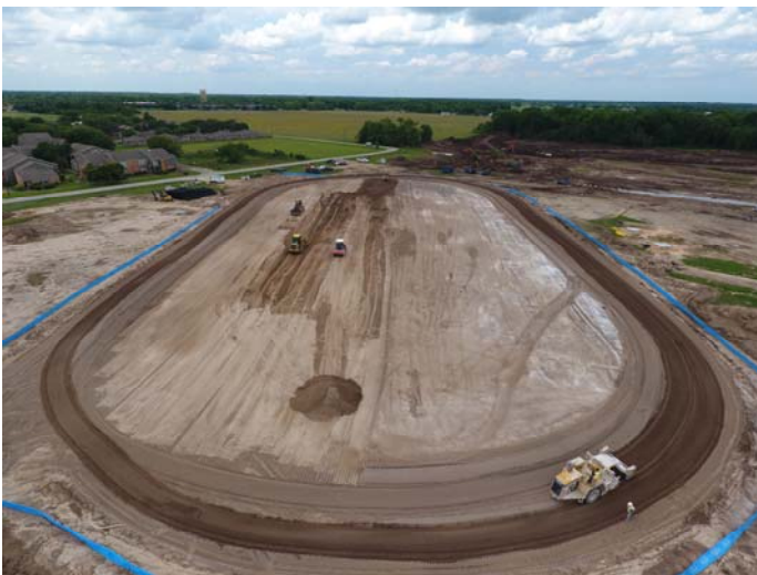
17. Lime stabilization of track
