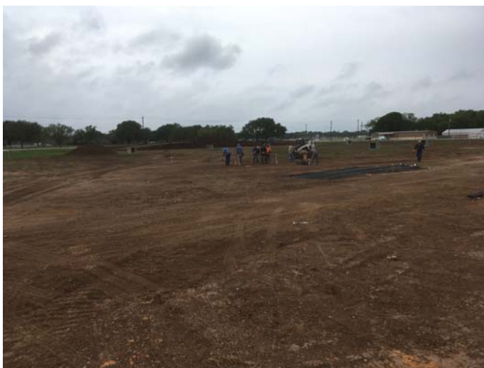
5. Site fab of drilled footing reinforcements
