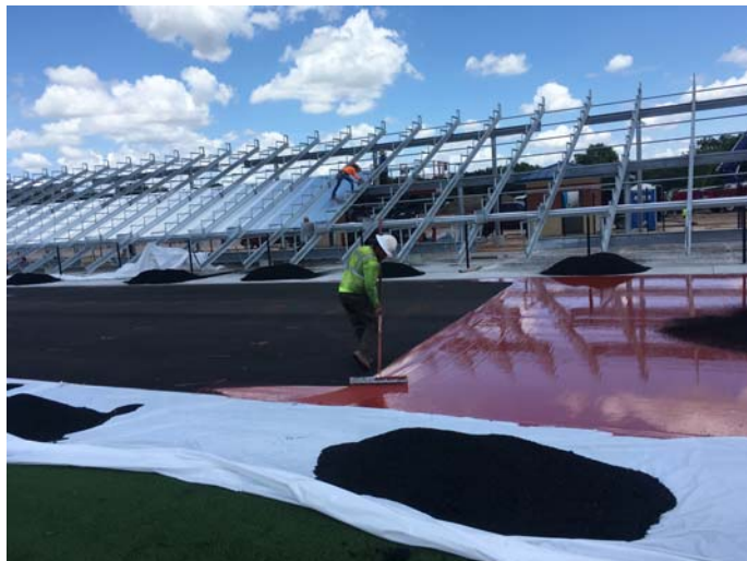
15. Track surfacing installation
