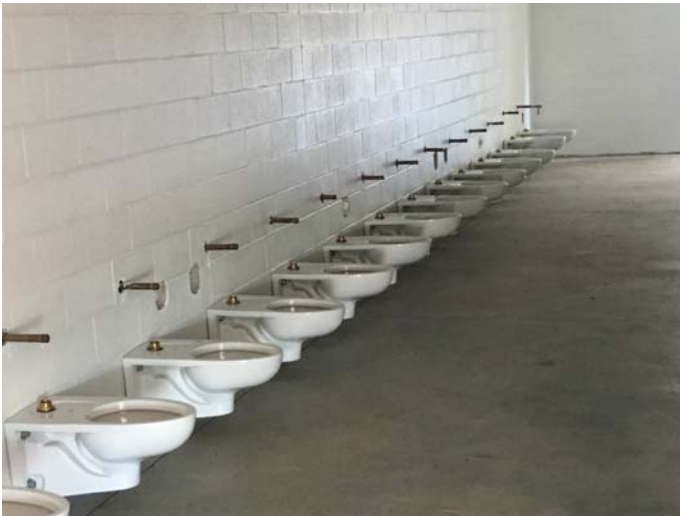
13. Water closet installation at women's restroom
