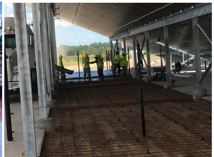
16. Concrete paving at home grandstands
