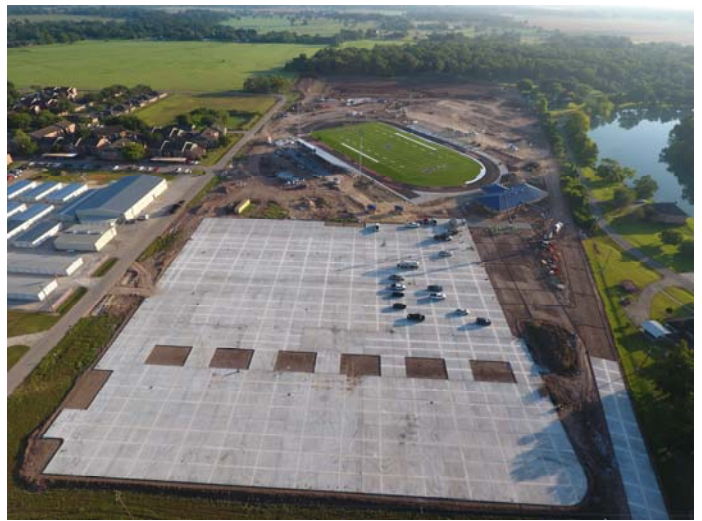
4. Concrete at home parking area
