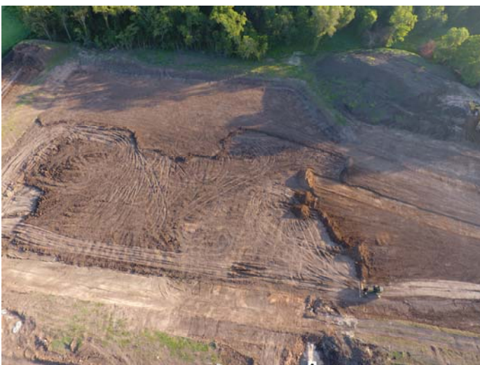
5. Final grade at detention area
