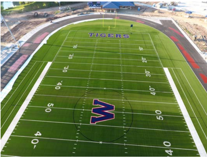
3. View of turf field at south end zone
