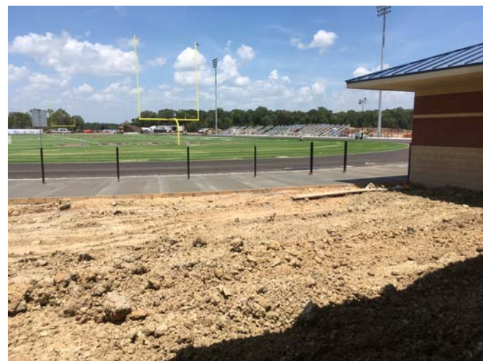
12. Concrete sidewalks at track perimeter
