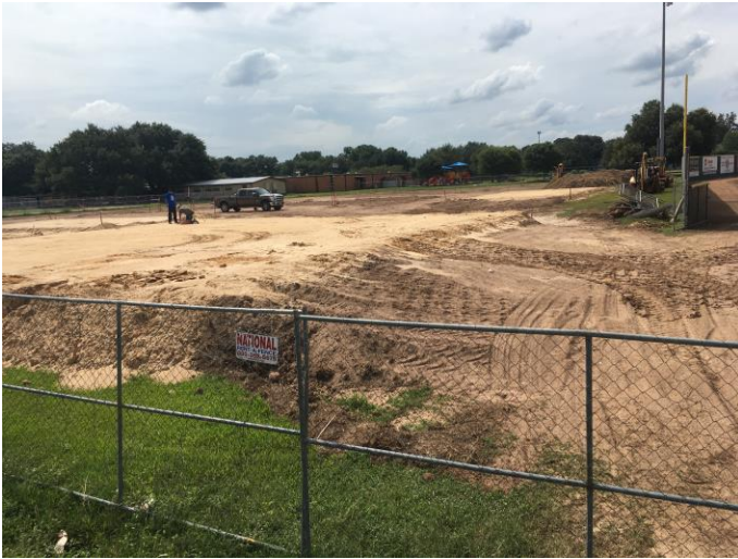
1. Select fill at concessions building pad
