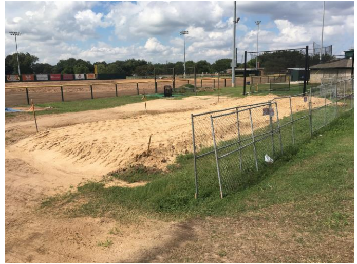
2. Select fill at entry building pads
