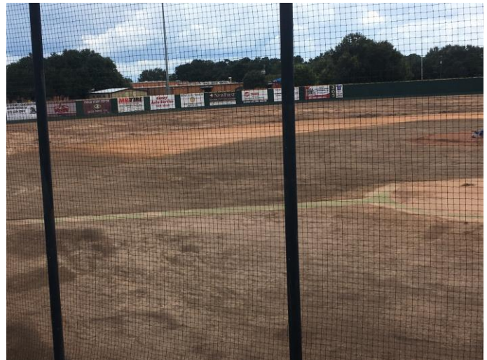
4. Removal of vegetation at baseball field
