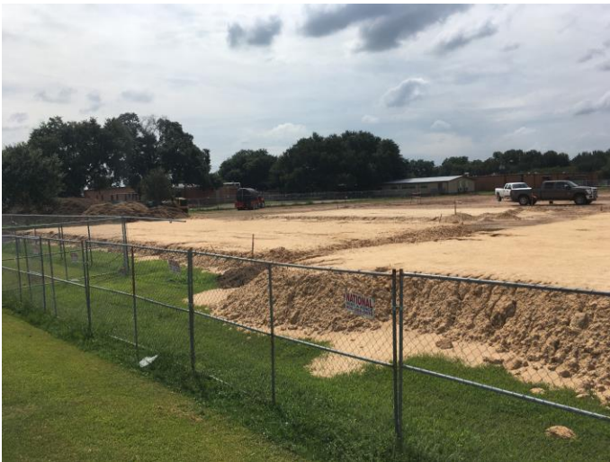
3. Select fill at batting cage building pad
