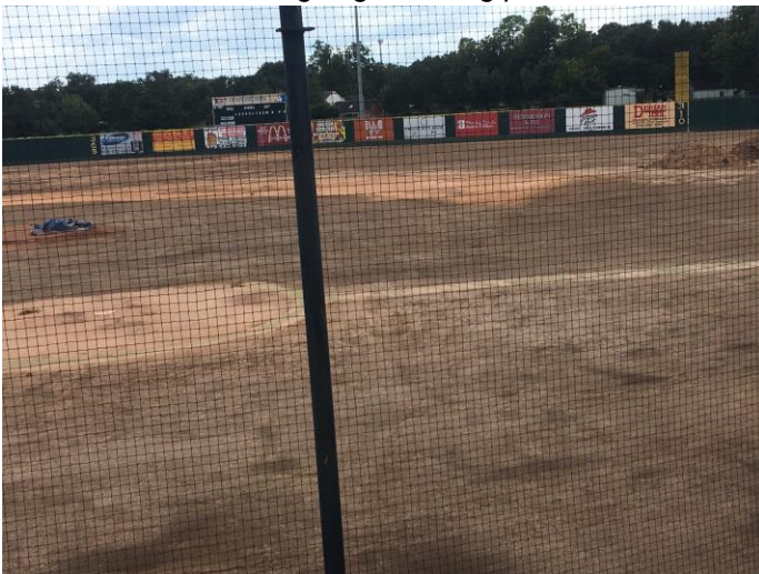
5. Removal of vegetation at baseball field
